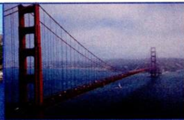
the Golden Gate Bridge (USA)
